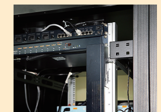
5. Z bracket, mounting style 2
